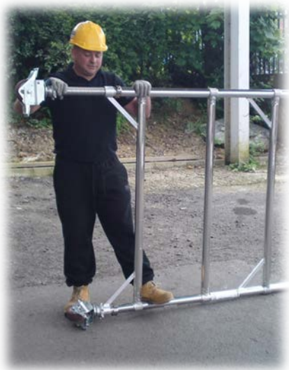
1. Insert 2 legs and castors into each frame.
