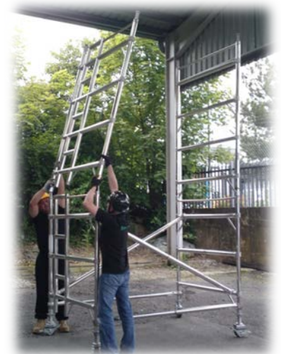
4. Add next level frames – according to your kit list.
