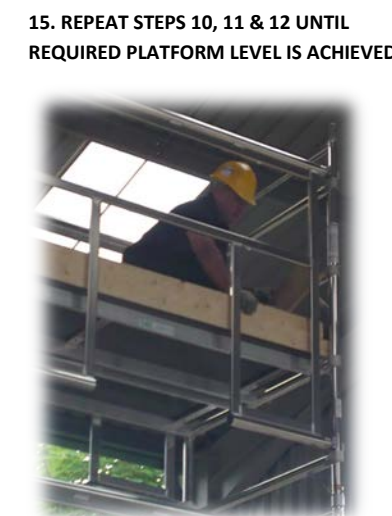
16. Fit toeboards in the correct position.
