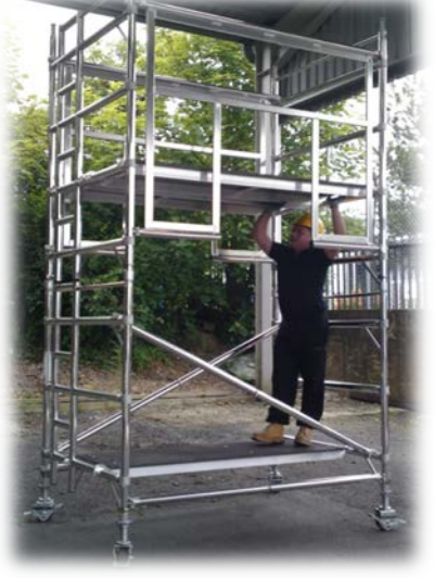
8. Position the trapdoor platform to the appropriate rung (Trapdoor facing the ladder section) 1 rung above the bottom section of the AGR frames.
