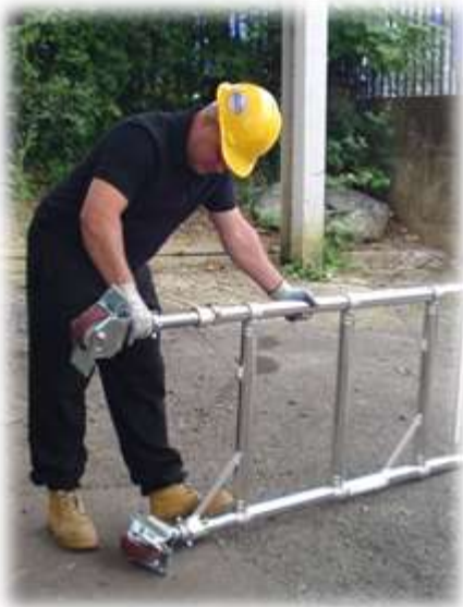
1. Insert 2 legs and castors into each frame.
