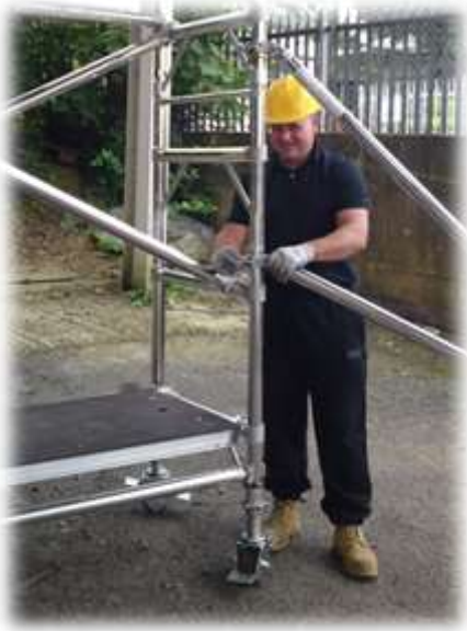
9. Secure stabilizers as soon as possible to increase tower stability.
