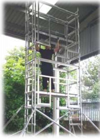
14. Remove the temporary trapdoor platform and position on the appropriate rung (Trapdoor facing the ladder section) 1 rung above the bottom section of the AGR frames.
