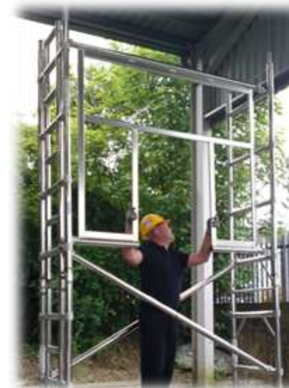
7. Standing on the platform with the green label facing you, position the 1 st pair of AGR frames to the vertical members above the rungs in the required position, as shown.
