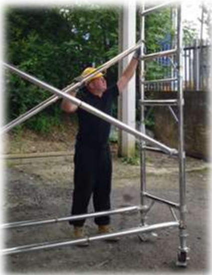
5. Add 2 diagonal braces, from the 2nd to 4th rung as shown.
