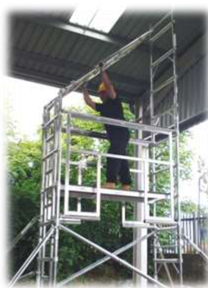
11. Add 4 rung frames, ensuring that the ladder is continuous.
