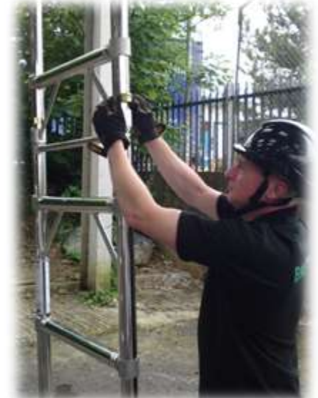
4. Engage Interlock Clips.
