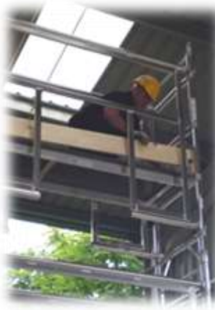
16. Fit toeboards in the correct position.
