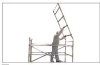
To add further frames, stand on platform ensuring the ladder frames are in line.
