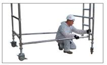
Fit in 2 horizontal braces to the vertical member of the frames, as low as possible, below the 1st rung. All horizontal braces fit on from inside the tower facing out.
