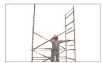
Klik in diagonal braces to continue in a regular pattern. Double Width towers always have diagonal braces either side of the tower opposing each other as illustrated.
