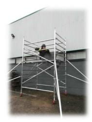
8. Access internally through the trapdoor and sitting with your feet on the rungs below, fit the mid and top handrails to form a safe guardrail to the 2nd and 4th rungs above the platform.
