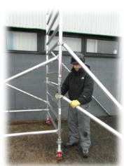
adjusting the leg nuts as required and secure stabilizers as low down as possible to increase tower stability, adjust according to the guide for
