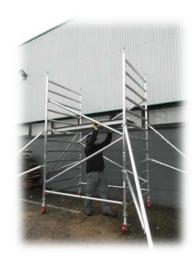
7. Fit trapdoor platform onto the rung above where the braces meet.
