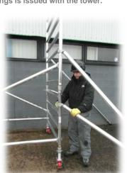
5. Level base using a spirit level as a guide by larger towers or to overcome obstacles.
