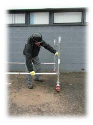
2. Fit 2 horizontal braces to the vertical member of the frames, as low as possible, above the 1st rung and lock the castors.
