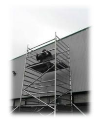
13. Access internally through the trapdoor and sitting on the fixed deck with your feet on the rungs below, fit the mid and top handrails to form a safe guardrail to the vertical tube above the 2nd and 4th rungs.
