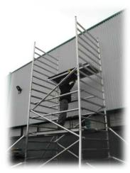
11. Fit 1st working level platform over to one side, 1 rung above the brace hooks.
