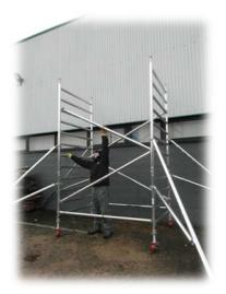
6. Fit 2 diagonals continuing the run, as shown. Even Metre Towers: Add 2 further diagonals continuing the run.
