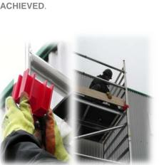
14. Fit red clips and toeboards in the correct position ensuring trapdoor opens freely.
