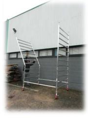
3. Add 1st set of 8 rung frames and engage the interlock clips
