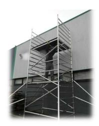
Fit 2nd working level platform alongside the other platform one rung above the brace hooks.
