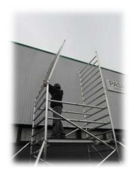
9. Add next set of 8 rung frames and engage the interlock clips.
