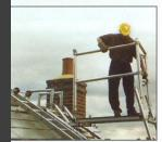
Fit handrail and engage interlock clips.
