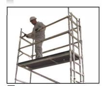
Dismantling is the reverse of assembly except to remove guardrail braces. Unclip the far end hooks and then from a sitting position through the trapdoor (3T) remove the guardrail braces. Do not remove the handrails whilst standing on the platform; this would put you at risk.
