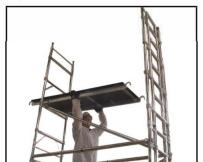
Facing the plain frame, fit a trapdoor platform on appropriate rung\* over the brace hook as near to the frame vertical as possible, trapdoor to ladder frame end (\*see base set up Fig 1 for guide).
