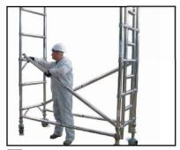
Facing the plain frame fit 1 diagonal to the bottom rung as close to the right hand frame vertical as possible. Facing the ladder frame fit 1 diagonal to the bottom rung as close to the ladder as possible.
