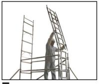
To add frames, stand on platform and offer frame up to the spigots ensuring ladder runs continuously.
