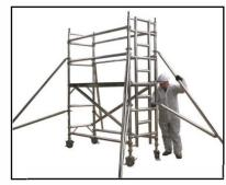
Secure stabilizers as soon as possible to increase tower stability, the lower arm as close to horizontal as possible.
