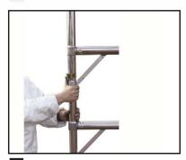
After adding frames, engage interlock clips.
