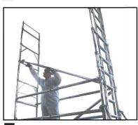
Fit the diagonal braces to continue in a regular pattern from rung to rung except when interrupted by an intermediate trapdoor platform.
