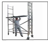
Facing the ladder frame, fit a trapdoor platform on appropriate rung\* inside the brace hook as near to the ladder as possible (\*see base set up Fig 1 for guide).
