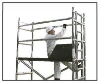
From a sitting position through the trapdoor (3T) fit four horizontal braces to the frame verticals above the rungs pushing from inside to out.
