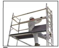
From a sitting position through the trapdoor (3T) fit four horizontal braces to the frame verticals above the rungs pushing from inside to out.
