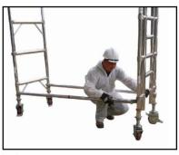
Fit in 2 horizontal braces to the vertical member of the frames, as low as possible, below the 1st rung. All horizontal braces fit on from inside the tower facing out
