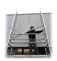
9. Fit 2 diagonal braces running in opposite directions starting from the rung in between the guardrail braces.
