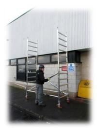
4. Fit 2 diagonal braces running in opposite directions on either side of the 1st rungs.
