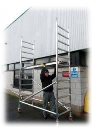
5. Fit trapdoor platform onto the 7th rung, leaving one rung clear between it and the lower braces. Level base using a spirit level as a guide by adjusting the leg nuts as required.
