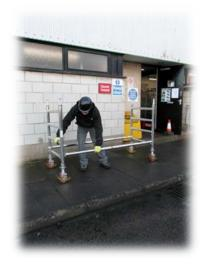
2. Fit 2 horizontal braces to the vertical member of the frames, as low as possible, above the 1<sup>st</sup> rung and lock the castors.
