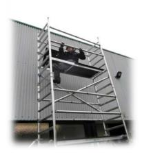
11. Access internally through the trapdoor and sitting on the fixed deck with your feet on the rungs below, fit the mid and top handrails to form a safe guardrail to the vertical tube above the 2nd and 4th rungs.
