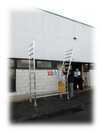
3. Add 1st set of 8 rung frames and engage the interlock clips.
