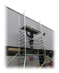
10. Fit next trapdoor platform 1 rung above the brace ends.
