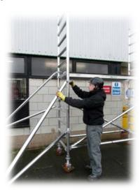
Secure stabilizers as low down as possible to increase tower stability, adjust according to the guide for larger towers or to overcome obstacles.
