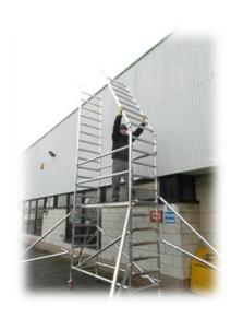
8. Add next set of 8 rung frames and engage the interlock clips.
