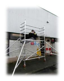
7. Access internally through the trapdoor and sitting on the fixed deck with your feet on the rungs below, fit the mid and top handrails to form a safe guardrail to the vertical tube above the 2nd and 4th rungs.
